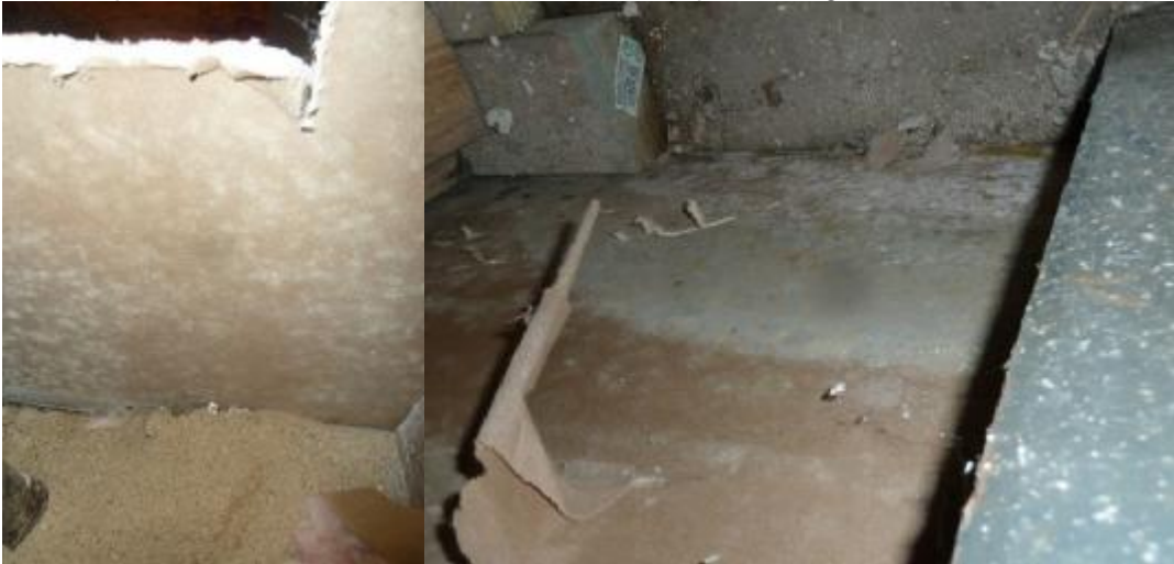
Mold at E wall, behind/left of furnace; stains at bottom of stairs; mold below access panel for main water valve; mold at plumbing cleanout area near bath
