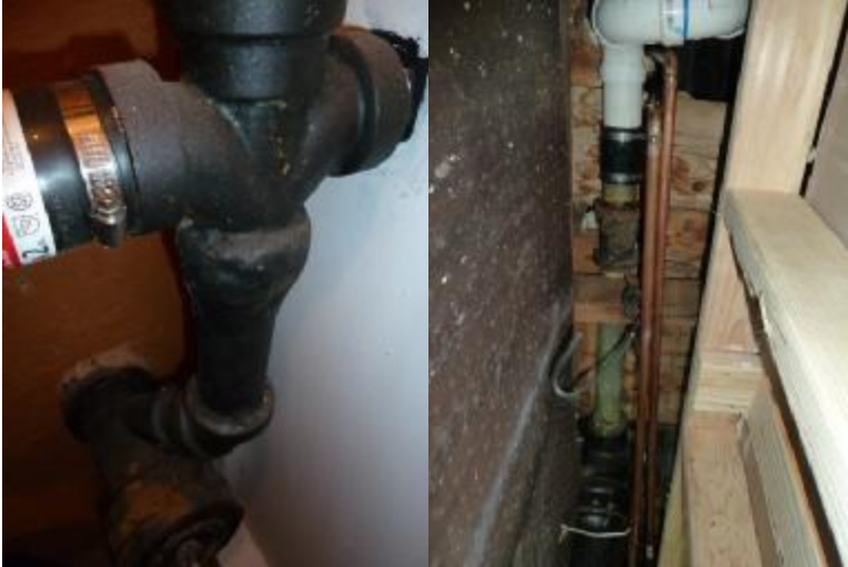
Patching betw. pipes, site of odor; note older piping being re-used, under bathtub; 1.5" not proper 2" vent for ejector; DW enters drain on sewer side
