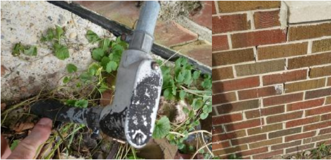
Garage is served by thinwall elec. conduit, not rigid conduit; cracking where garage meets landscape wall; interior and gap betw. roof and fascia
