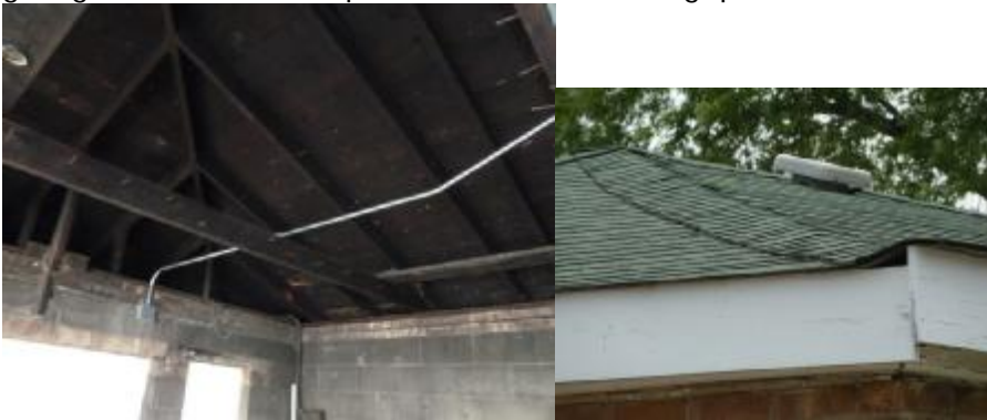
Garage is served by thinwall elec. conduit, not rigid conduit; cracking where garage meets landscape wall; interior and gap betw. roof and fascia
