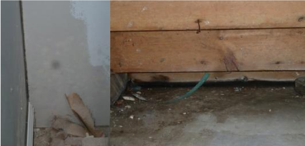
Mold at E wall, behind/left of furnace; stains at bottom of stairs; mold below access panel for main water valve; mold at plumbing cleanout area near bath
