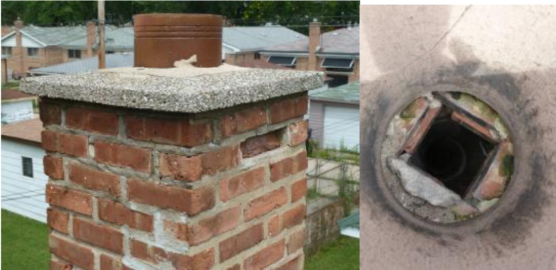
Chimney in & out
