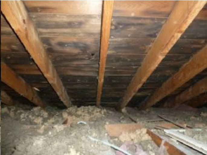
patched hardwood; poor insulation, dark spots indicating mold in attic
