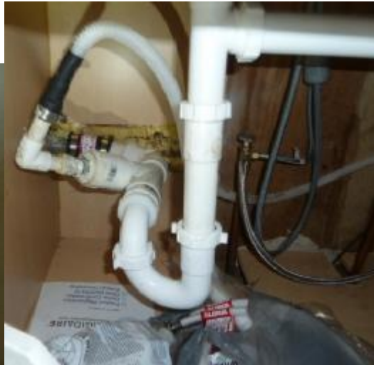
Patching betw. pipes, site of odor; note older piping being re-used, under bathtub; 1.5" not proper 2" vent for ejector; DW enters drain on sewer side
